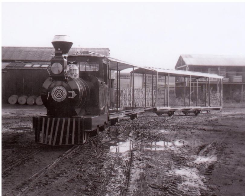
Another view of 22224 in Motor Rail's yard, but this time with two coaches. This photograph suggests the coaches were supplied as they are seen here - as frames complete with running gear and roofs, but with no floors or seats. These were added by Wicksteed.
